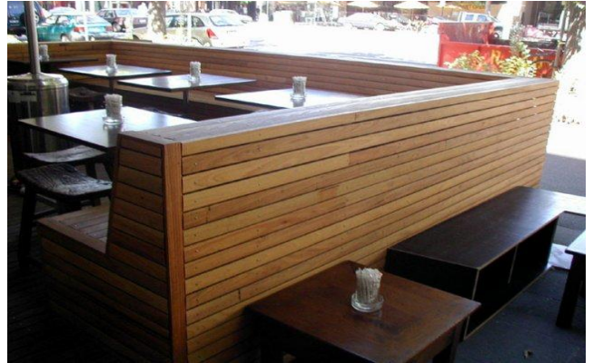
Yellow Stringybark decking(80 x 19) used for seating.
