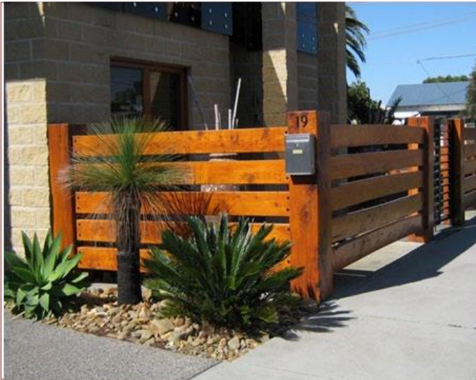
200x200 Posts and 150 x 38 Board Dressed Cypress Fence
