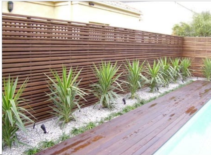
Stained Silvertop ash screen boards (Alternating sizes 75 x 25 & 50 x 23)
