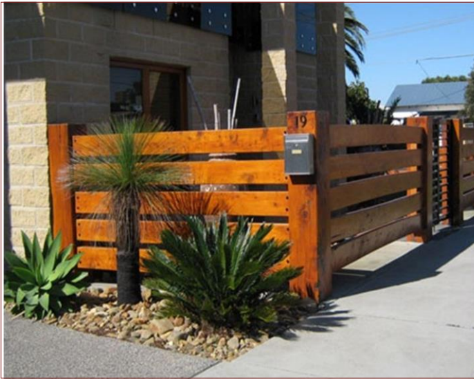
200x200 Posts and 150 x 38 Board Dressed Cypress Fence
